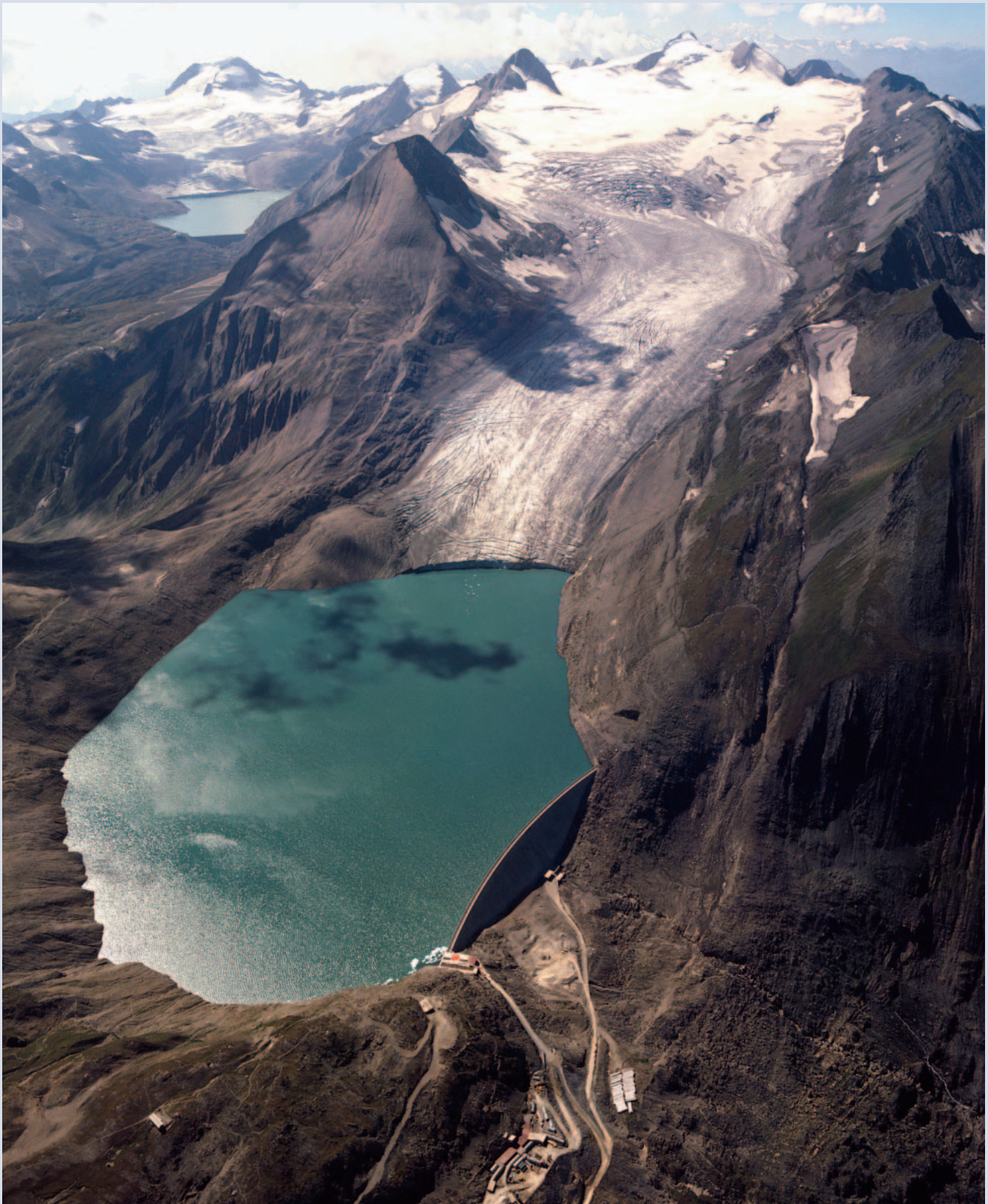
FIGURE 1 The Gries dam in 1973, fed by the approximately 5-km-long Gries Glacier near Ulrichen, Canton of Valais. Since this photo was taken, the glacier has lost over 370 m. (©Luftbild Schweiz)
